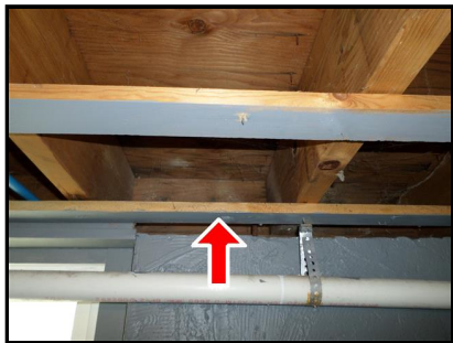
8.5 Item 1(Picture) perimeter sill no insulation
