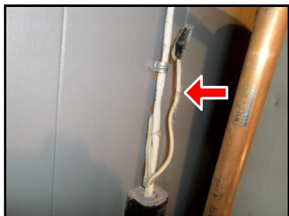
11.2 Item 1(Picture) un-secure wire
