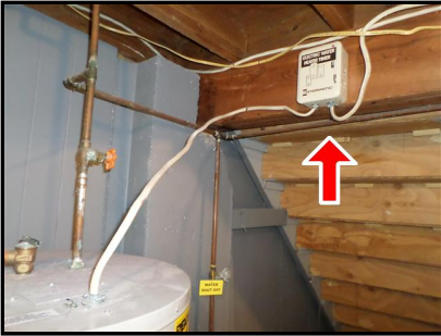
10.3 Item 1(Picture) hot water heater timer
