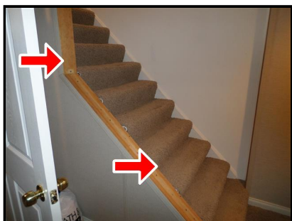
6.3.C Item 1(Picture) missing handrail
