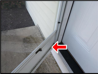
2.0 Item 1(Picture) missing door closer
