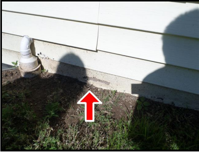
2.4 Item 1(Picture) damaged vinyl siding
