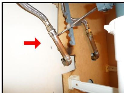
5.4 Item 1(Picture) No shut off valves
