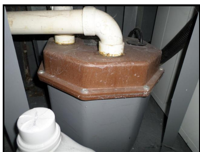
9.7 Item 1(Picture) sewer ejector pump
