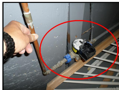
11.1 Item 3(Picture) missing jumper cable
